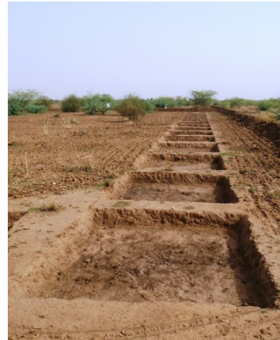
Series of Chauka tanks being built
